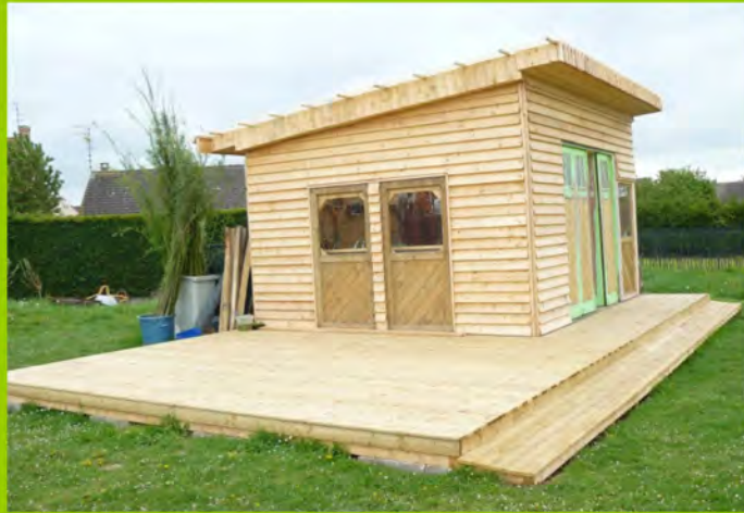
Abri convivial (Eco-construction)
